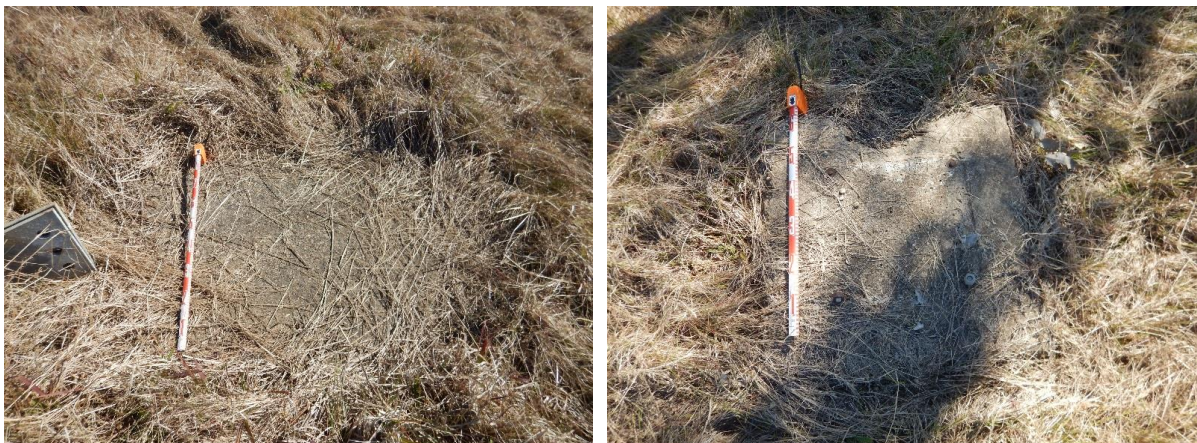
Figure 4: Concrete tower footings, 2016 (Source: Artefact Heritage)
